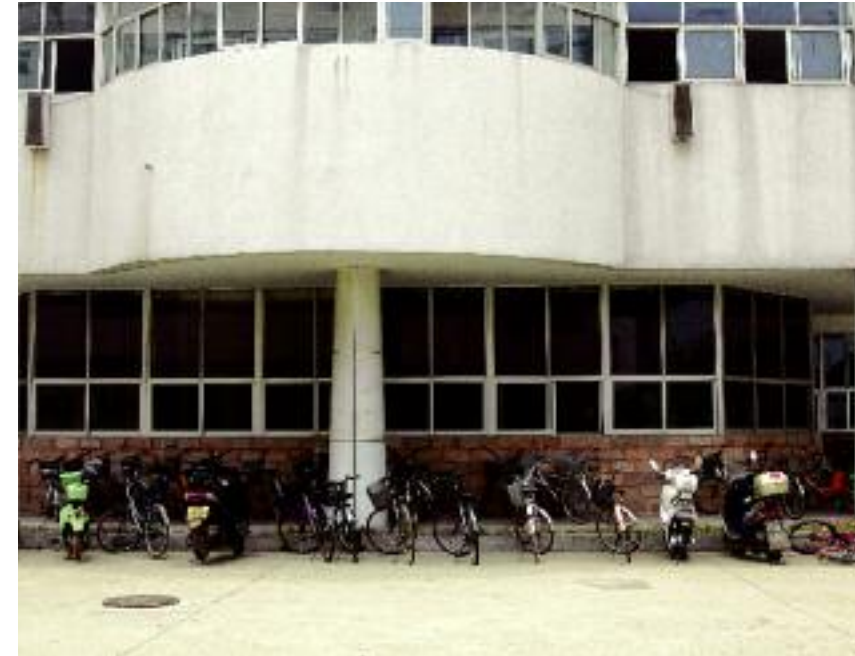
Students park their bikes outside the academic buildings where their classes take place at Anhui University.
